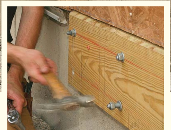
Drill the concrete. Use a rotary hammer or hammer drill with a 1/2-in. masonry bit to drill into the concrete at each hole. Spin the nut onto the bolt before setting it with a hammer. This eliminates the problem of screwing nuts onto damaged threads.
