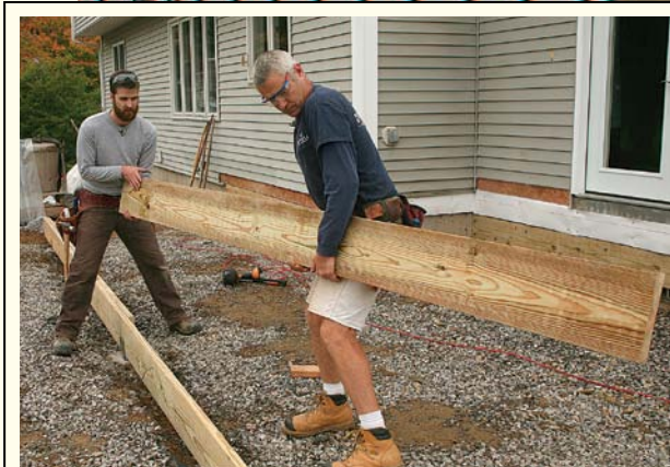
Build the beam in place. This two-ply beam is made up of four 2x10s. The two butt joints are located directly on separate post bases.
