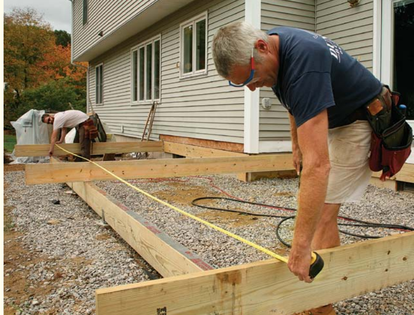
Parallel sides. After checking for square, make sure that the end joists and center joist are parallel.
