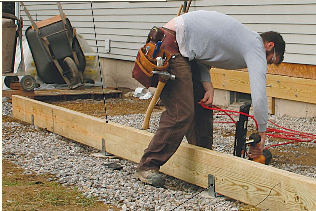
Build the beam in place. This two-ply beam is made up of four 2x10s. The two butt joints are located directly on separate post bases.
