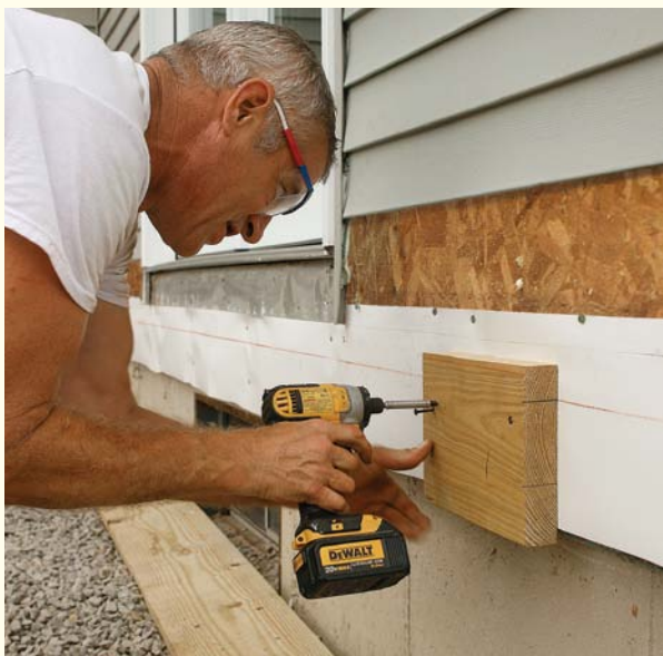
Lay out and drill. Measure and cut 2x10s to length for each ledger, then use a framing square to lay out joist positions and the locations of the 1/2-in. expansion bolts.
