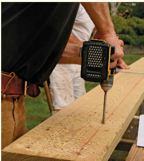
Lay out and drill. Measure and cut 2x10s to length for each ledger, then use a framing square to lay out joist positions and the locations of the 1/2-in. expansion bolts.
