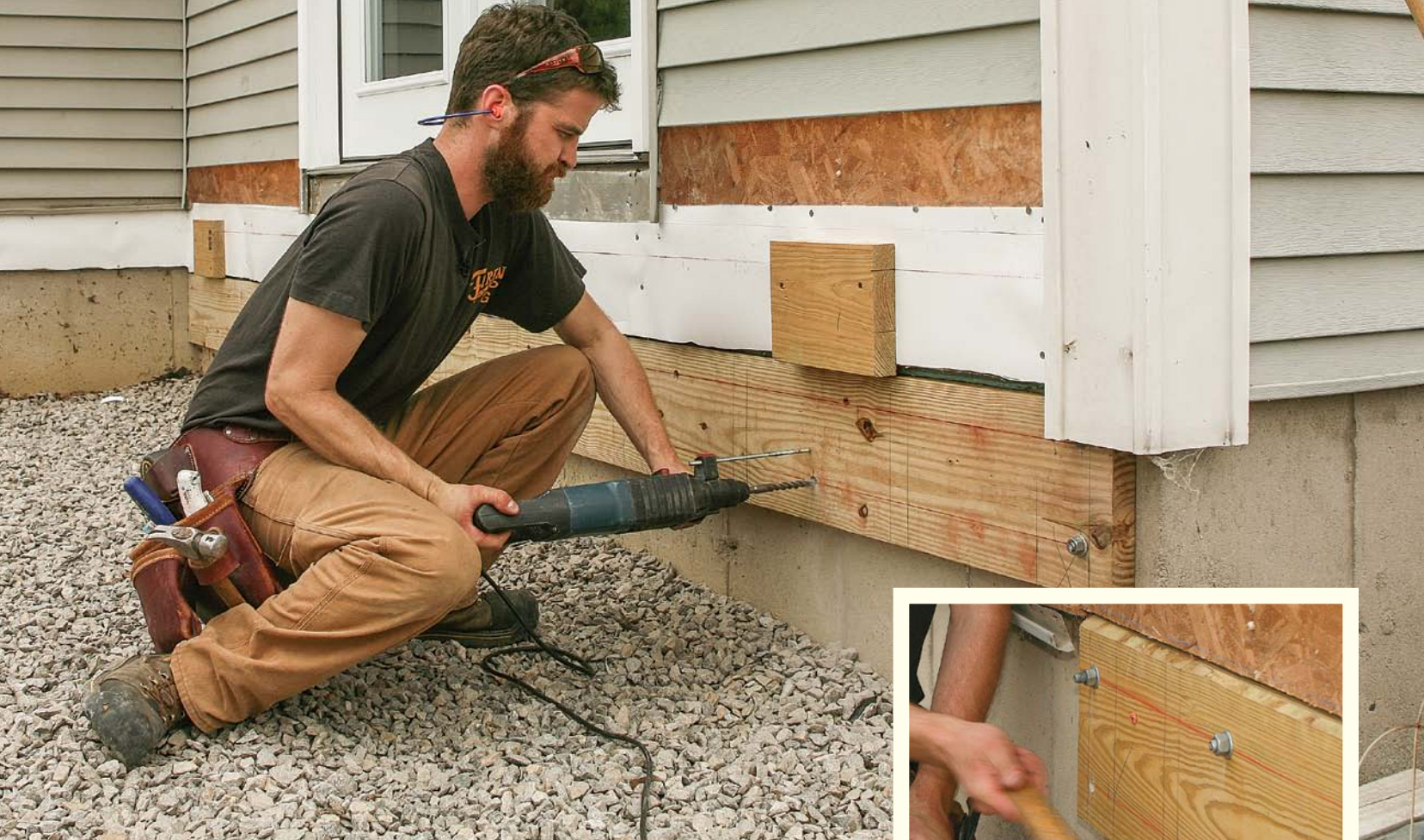
Drill the concrete. Use a rotary hammer or hammer drill with a 1/2-in. masonry bit to drill into the concrete at each hole. Spin the nut onto the bolt before setting it with a hammer. This eliminates the problem of screwing nuts onto damaged threads.
