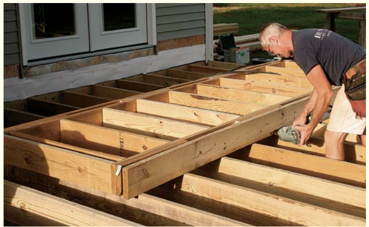
Extra padding. As on the main deck, the platform's decking perimeter of wider 5/4x6 boards requires blocking along the front and back.
