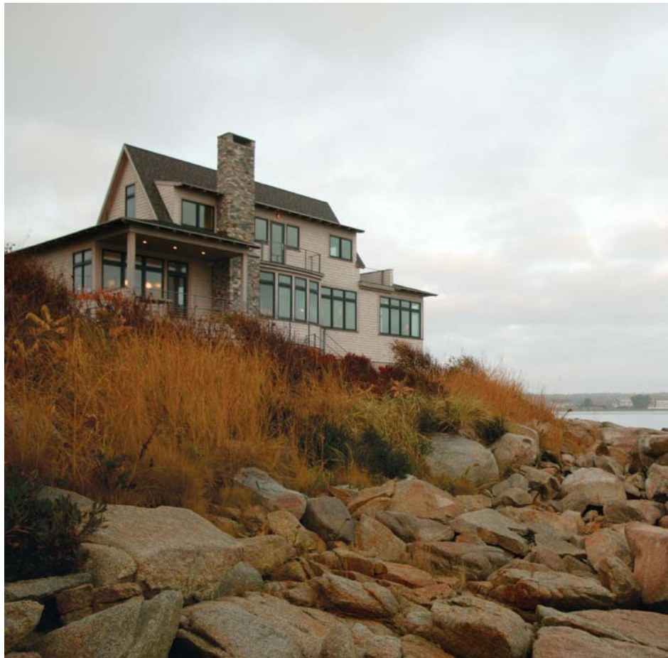
Banking on the view. Taking advantage of the ocean views to the northeast required a conscious decision to accept the energy penalty the multiple windows would incur.
