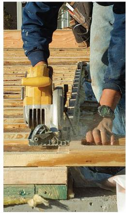
After aligning the joists, snap a chalkline and cut them to length in place. Beware of anchor bolts lurking below when making this cut.
