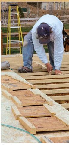
Sheathe your way over to where blocking is needed. Do not walk across unstable joists or work from a ladder below the floor. Sheathe over to the beam, then add the joist blocking.
