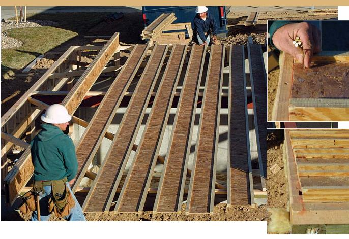
Position the square ends of each joist to the chalkline (the rim-joist line) and tack them into place along their 16-in. o.c. layout lines. Later, the 8d nail will act as a hinge when the joists are stood upright.
