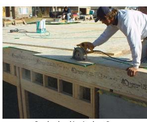
**Cut the sheathing in place.** Run sheets long at the ends, snap a chalkline, and cut off the excess. This process is faster and turns out a better floor than cutting each piece to fit.
