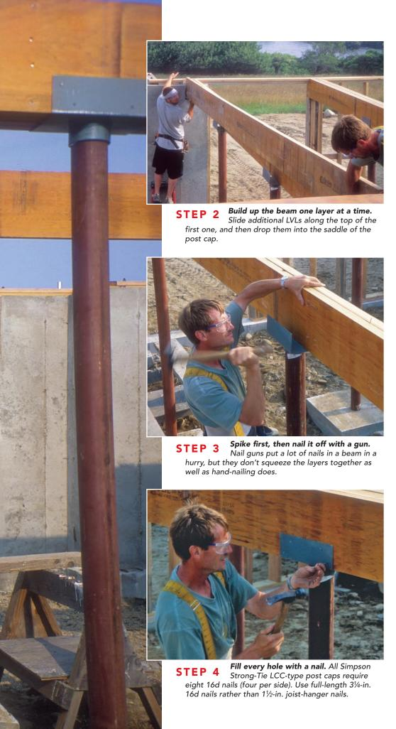
crane operator to set it in place for you, but you need to respect his time. Work quickly to cut the beam to length, and have the beam pockets ready to go. A chainsaw can make cutting big beams go faster.
