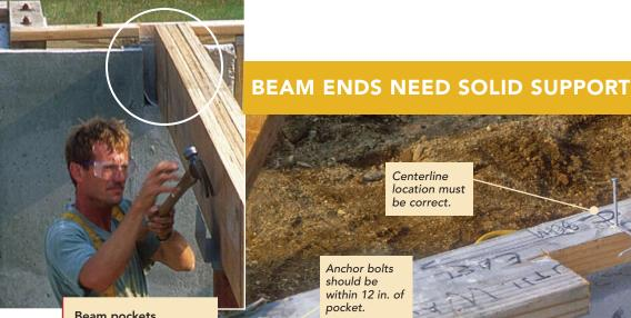
Beam pockets, whether formed or cut into masonry walls, need to be sized and detailed correctly. In a perfect world, accurate plans on-site before the foundation is poured would ensure a perfect pocket. The beam would sit on sill seal and be flush with the mudsill.
