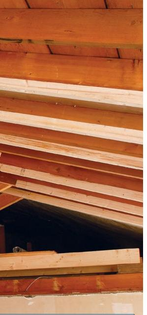
joists to the plates; this process prevented the joist ends from splitting. Once the nails had been removed, the strapping and the joists would provide much of the lumber needed to frame the new ceiling.
