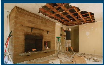
Protect the floor during demolition. Hardwood floors are protected by moving blankets under a layer of 6-mil plastic, which also makes cleanup easier. The old 16-in.-wide gypsum board and ½-in. plaster are easiest to remove by pulling down along the panel edges. Pieces usually break into 16-in. by 8-ft. slabs. Careful demolition also preserves strapping and rafters for later use.
