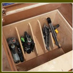
Close to the wall. This lockbox location makes it hard for a thief to get at the hinges, a vulnerable point on many boxes. I lag-screw the box through the subfloor and into the floor framing.
