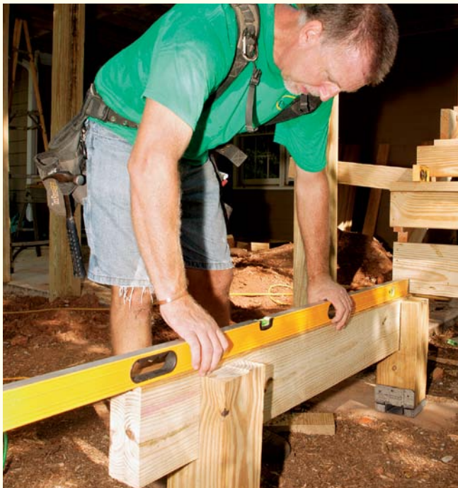
Angle brackets Simpson A35Z or similar
