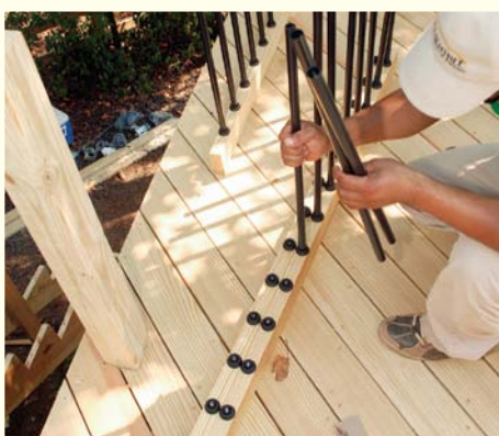
Center the baluster cups. Screw down the cups to the rails in pairs so that the balusters have the same spacing on the top and on the bottom.
