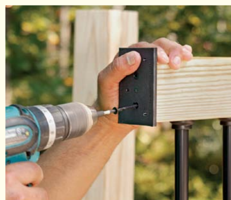
Connect railings to posts with brackets. After the balustrade is assembled, screw brackets onto the railing ends. Then screw the brackets from the opposite side onto the posts to attach the assembly.
