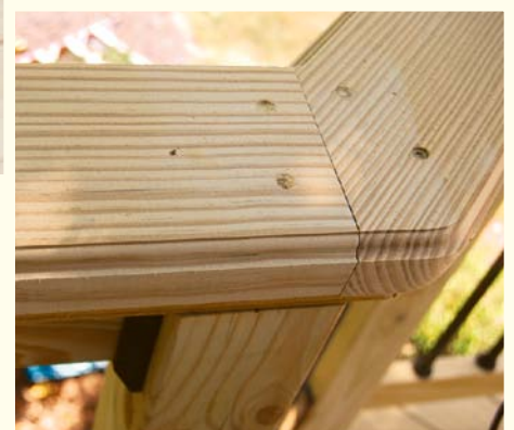
Tie everything together. Railing caps made from 2x6s connect each of the posts and add strength to the balustrade. An ogee profile routed onto the edges gives the rail a finished look.
