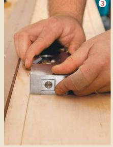
**Clean up the bearing surface.** Use the shoulder plane to smooth the dadoed area. Then turn it on its side, and square up the perimeter edges.
