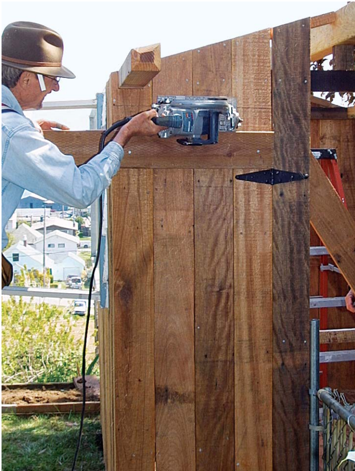
A saw cuts the top and bottom of the door.
