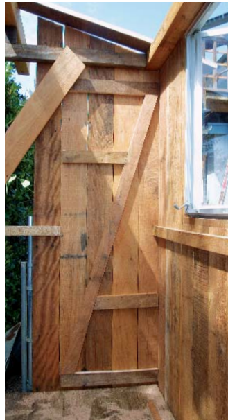
Bracing goes on the inside.
