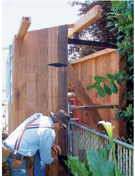
Hinges join the door to the jamb board.
