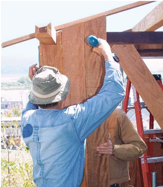
First, the wall boards are screwed in.
