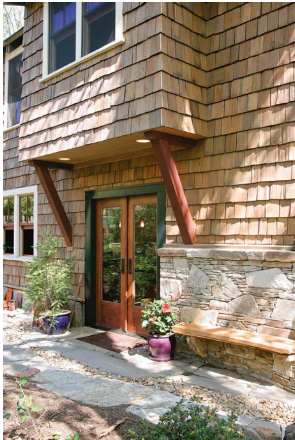
A short commute. The basement office has its own grade-level entrance. Double doors, brackets, and a sheltering bump-out lend a professional presence. Inside, the radiant-slab floor was finished inexpensively with concrete stain and sealer. Photos taken at C and D on floor plan.
