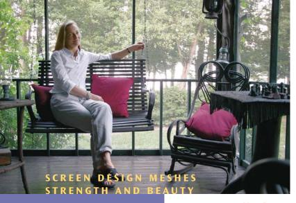
The basis for our porch design was both aesthetic and practical. The cedar log posts were chosen as a way to connect to the natural setting and were left untreated so they would weather to a natural gray patina. The framework between the posts supporting the screens is as slender as possible and painted dark green to blend with the foliage beyond.
