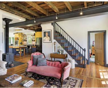
**Bold moves.** As with many remodels, improving this home's function meant finding a way to connect the kitchen with the living room. To get this done, we did two big things: removed the home's two masonry chimneys, allowing more flexibility in the rooms on both floors, and opened up the load-bearing wall between the original entry and living room using a steel I-beam.
