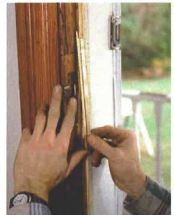
Bridging the lockset. If there isn't enough room to run interlocking strips past the lockset, a section of spring bronze weatherstrip covers the gap.
