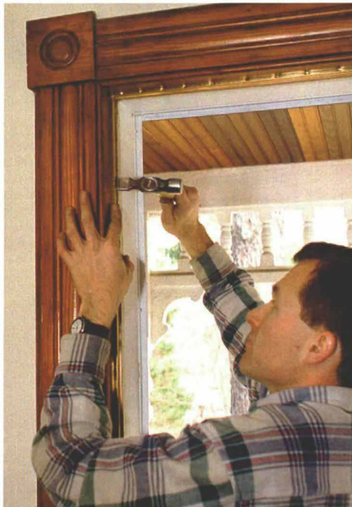
Bridging the lockset. If there isn't enough room to run interlocking strips past the lockset, a section of spring bronze weatherstrip covers the gap.
