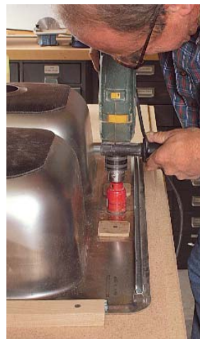
Finishing the hole from above reduces tearout. When the bit pokes through the laminate, flip it over and finish the cut from above. Screw cleats through extra faucet holes.
