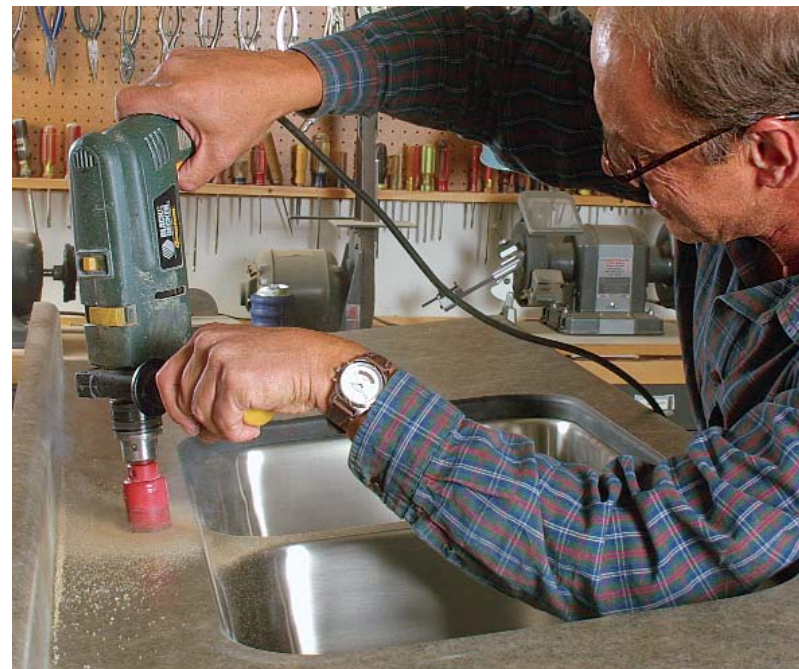
Finishing the hole from above reduces tearout. When the bit pokes through the laminate, flip it over and finish the cut from above. Screw cleats through extra faucet holes.
