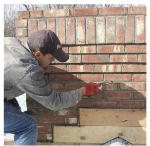
Strike the joints. After the mortar in the joints has firmed up, strike them smooth with a jointer tool. For a neat look, always strike the horizontal (bed) joints first, and then strike the vertical (head) joints.
