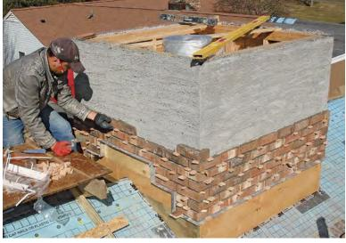
Stick the brick. Back-butter each piece of brick before sticking it to the scratch coat of mortar applied to the surface of the chimney box, using 3/8-in.-thick wood spacers to prevent the bricks from sliding down the chase as the mortar sets. For realistic-looking corners, be sure to order L-shaped corner bricks, which eliminate a tell-tale seam.
