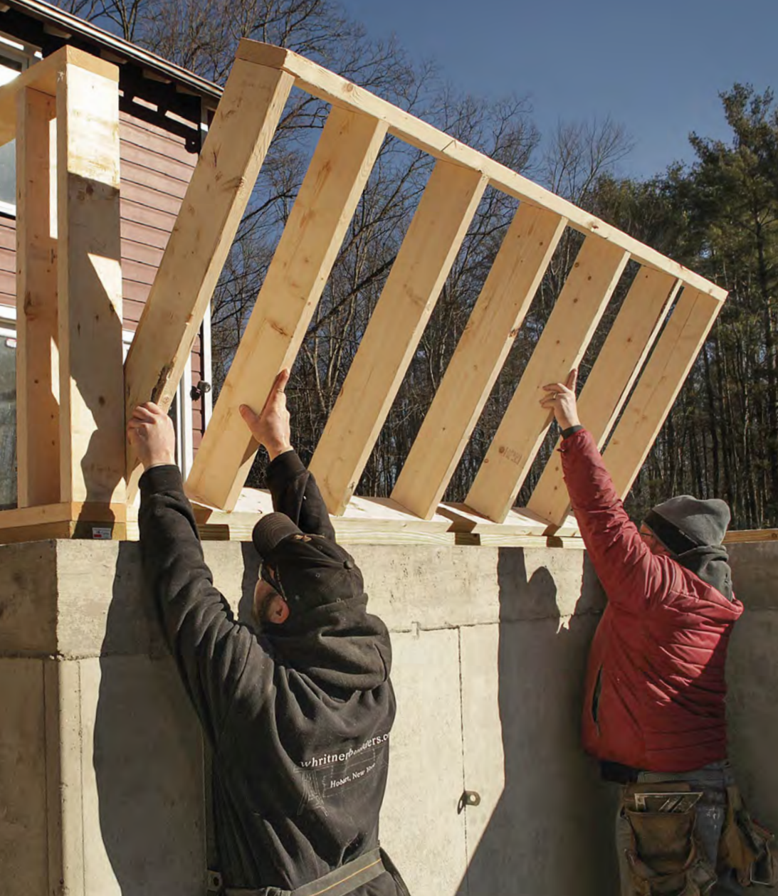
Tip 'em up. After lifting the cripple walls, tack them to the mudsill and to each other with 3-in. construction screws.
