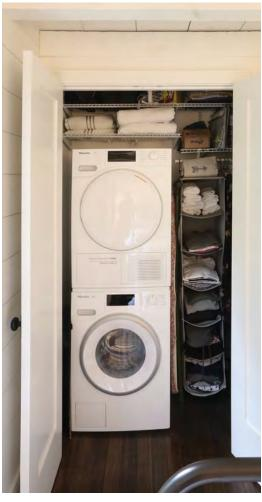
**STACK EFFECT** The Miele Stackable Compact washer and dryer easily tucks into the master-bedroom closet. The dryer is a condensing unit, so traditional venting isn't necessary, which makes placement within a small home much easier.
