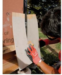
PUSH AND MARK To create a woven outside corner, use hand pressure to push a shingle into place at one side of the corner while using the other hand to mark the backside along the beveled backers. This first cut—which is on the undercourse—won't be seen, so it doesn't need to be perfect.
