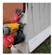
WEAVE UP THE CORNER Continue alternating the seams as you work upward. Water that penetrates a seam will get stopped by the face of the shingle behind it.
