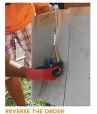
To cover the undercourse, follow the same sequence, but start the process on the opposite side so that once fastened, the corner joints are staggered, or woven.
