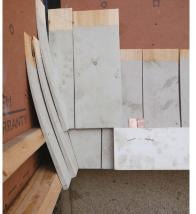
**INSIDE CORNERS ARE MUCH THE SAME** The concept of weaving flared shingles on an inside corner is the same as on an outside corner—change the overlap from one course to the next—except instead of holding a shingle in place to trace it, you have to rely on scribing to sneak up on a tight fit.
