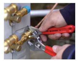
**No vacuum pump needed.** Precharged line sets with quick-connect fittings make it easy to install Mr. Cool Mini-Split ductless air-conditioning and heat pump systems without special refrigeration tools or training.
