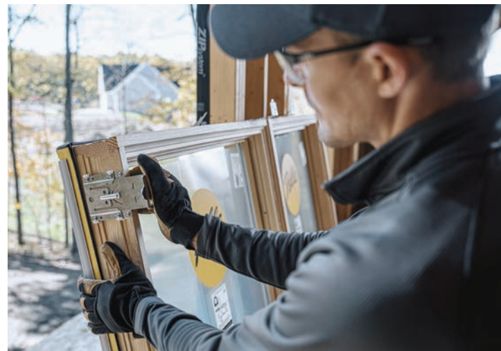
Stay inside. Pella's Steady Set windows install from inside the structure, using metal clips that fasten to the framed opening. A fold-out flange allows conventional flashing techniques.
