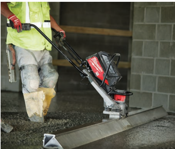
Gas-free screed. A 72v, 3-Ah battery powers Milwaukee's vibrating power screed for two hours when using a 12-ft. screed.
