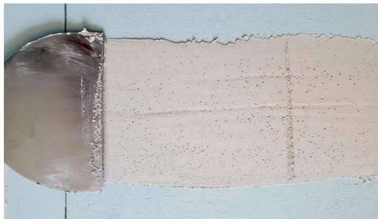
**Bubble buster.** Joint compound applied to painted surfaces often develops bubbles that complicate finishing. To fix the issue, apply a heavy coat of lightweight compound and let it dry for 30 minutes before smoothing it down.
