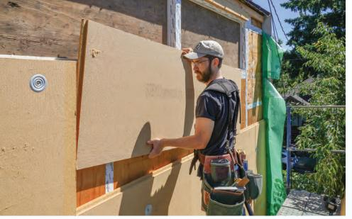
**WOOD FIBER** With similar characteristics to mineral wool, plus high compressive strength and a relatively low carbon impact, wood fiber is another option for CEI. Long available in Europe and gaining popularity with U.S. builders, these boards also have tongue-and-groove edges, which offer installation advantages. R-values are around R-3.5 per in.
